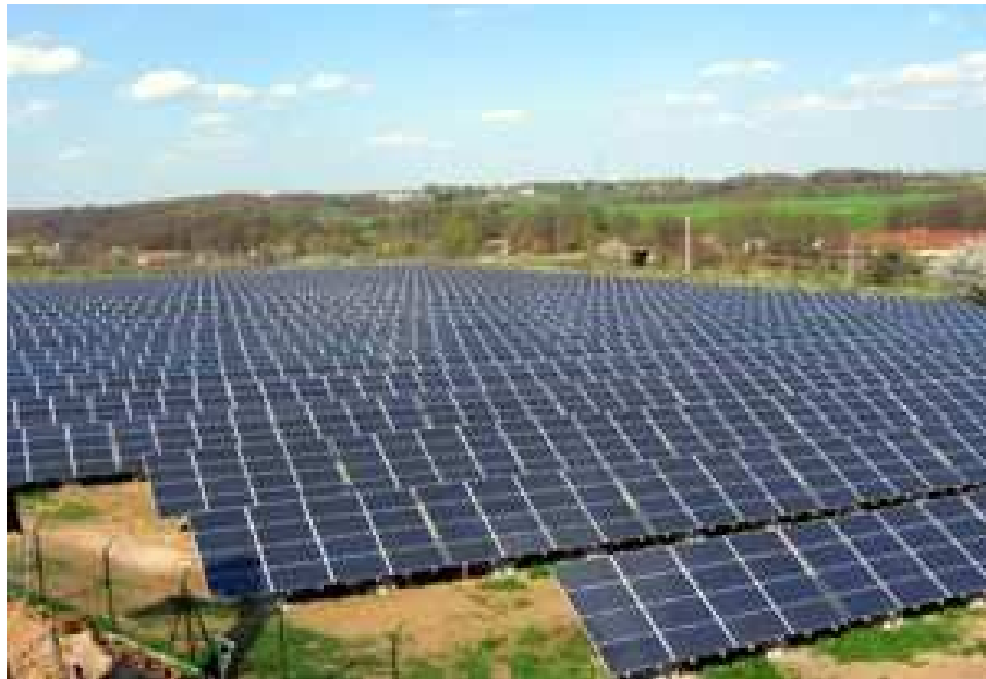
Picture 2: New energy system PV near Meerane
